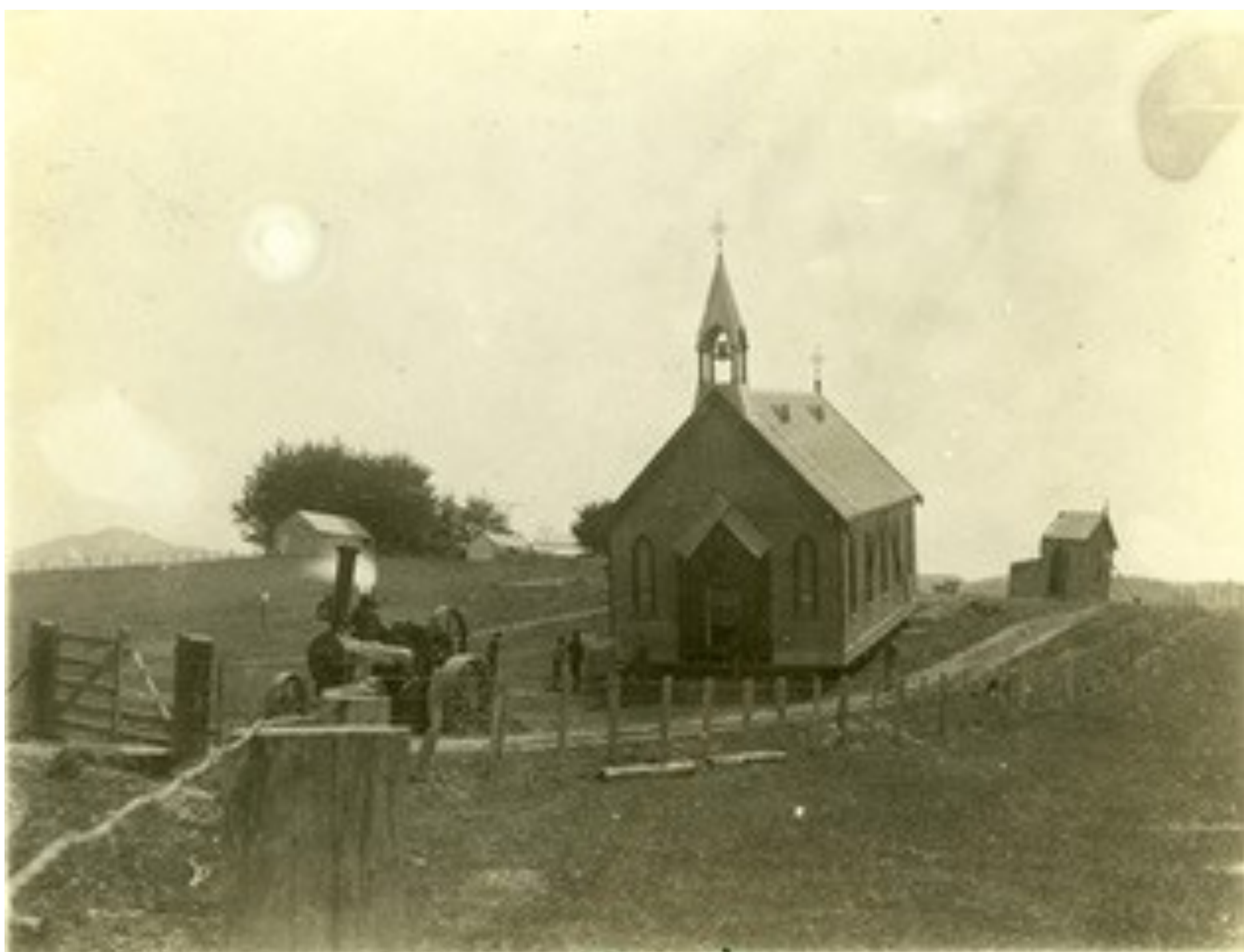
A traction engine pulling a church (minus vestry) down the hill before following the road to Owaka, Oct-Nov 1907.
